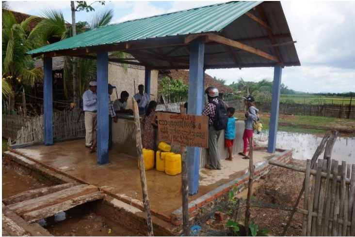
photo 7 New Built Village Water Supply Facility
