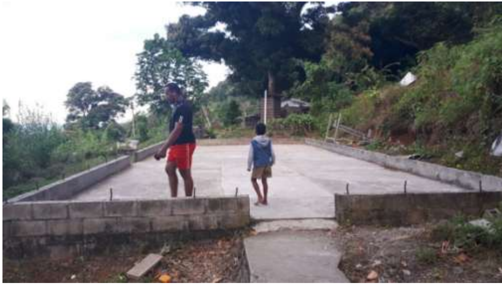
Figure 15: Charlie (left) at the community gym foundations, Baba.
